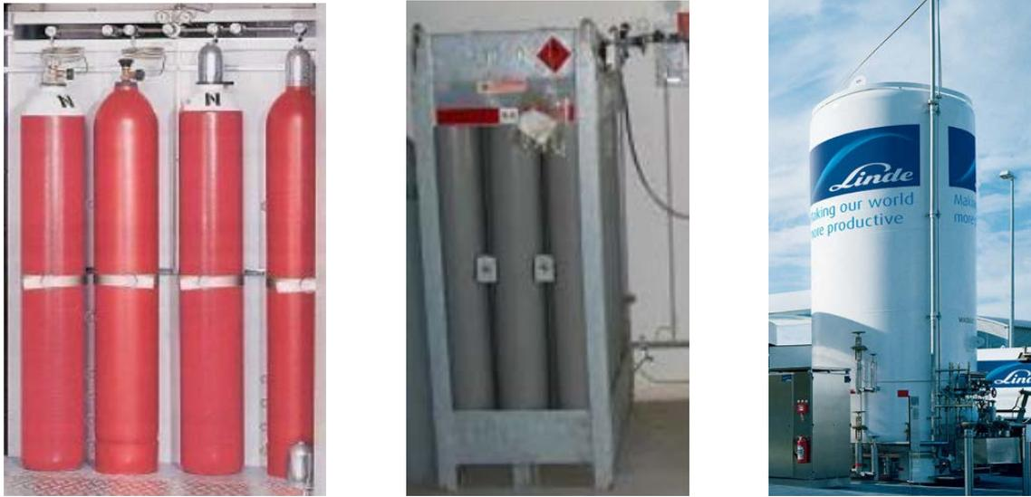
FIGURE 4: INDIVIDUAL CYLINDERS, A CYLINDER BUNDLE AND A CRYOGENIC STORAGE TANK
