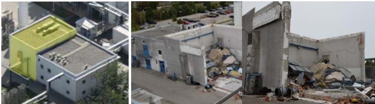
**FIGURE 2: HYDROGEN EXPLOSION IN A COMPRESSOR BUILDING**
